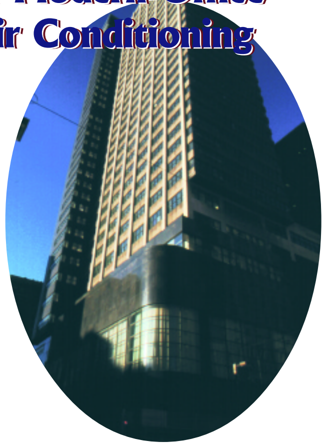
The PSFS Building in Philadelphia, completed in 1932, broke new ground in its architectural style and the concept of air conditioning.
